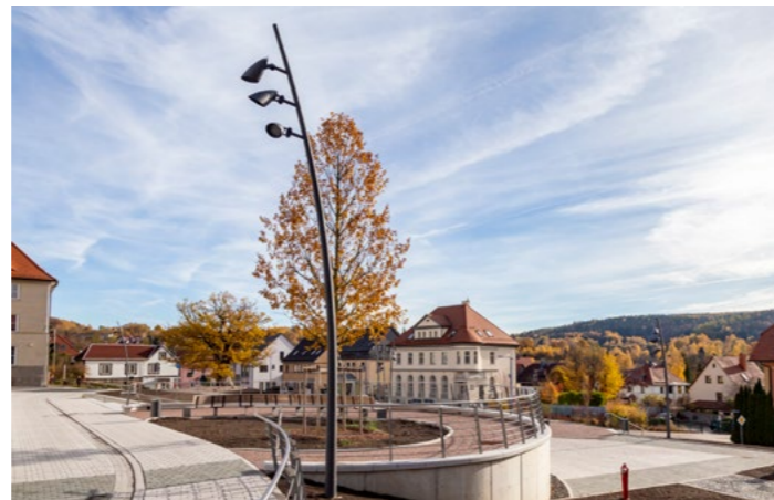
The new square offers a variety of utilisation possibilities – at different levels.
