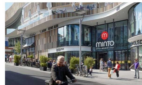
The FARO luminaires underscore the high-end overall impression of the Minto shopping centre.
