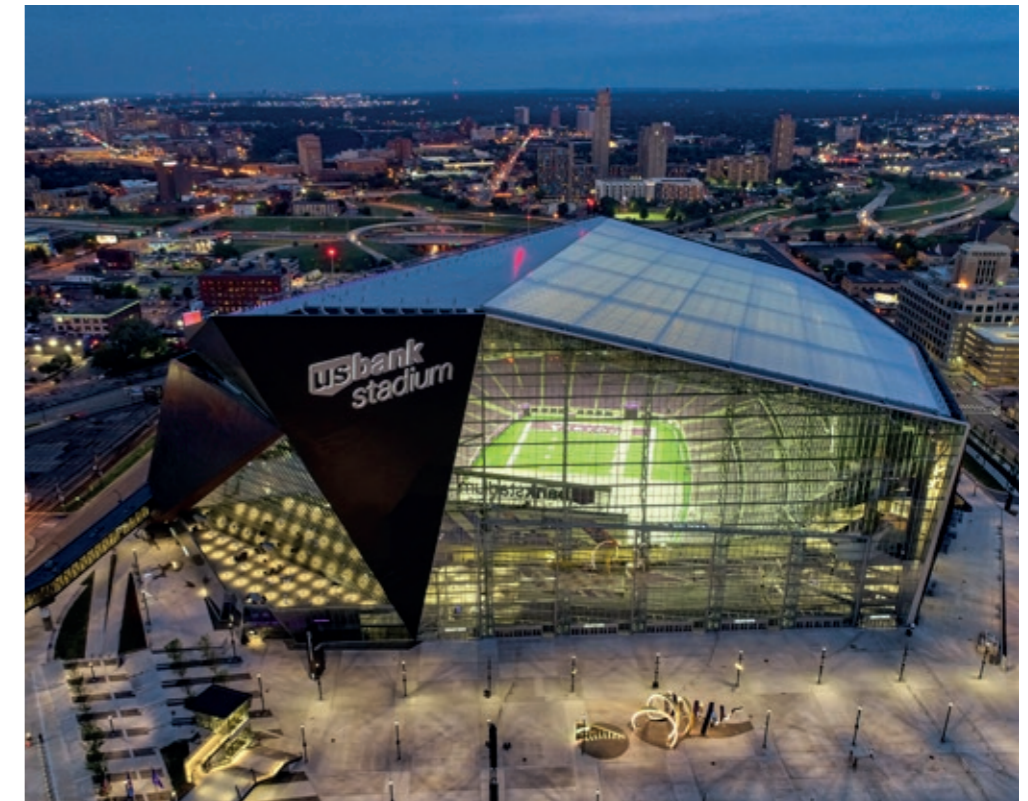
Imposing: The glass façade and the roof made largely of foil provide a light-filled stage. The outdoor area is lined with CITY ELEMENTS 230 at different heights.
