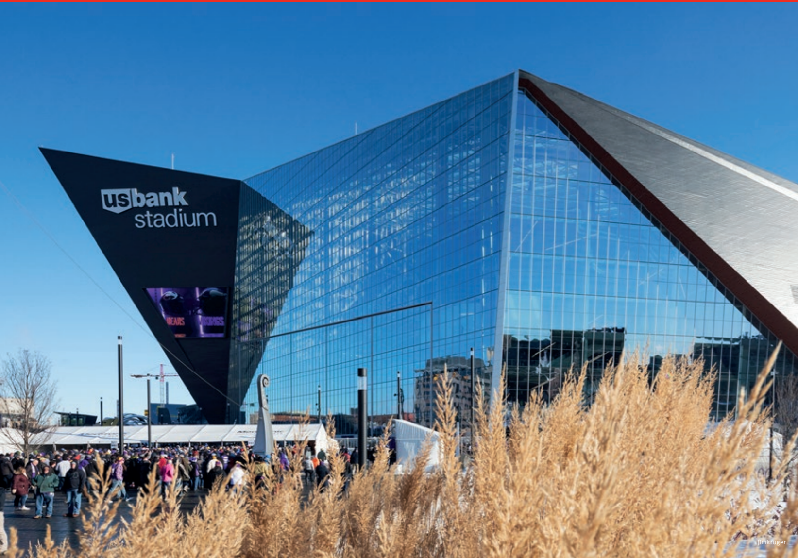
Impressive Architecture: The U.S. Bank Stadium with its huge glass façade attracts visitors magically. The multifunctional illuminating columns CITY ELEMENTS by Hess blend in with the outdoor space.
